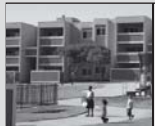
Cover: Plaza East, a 193-unit public housing development in San Francisco, California.
